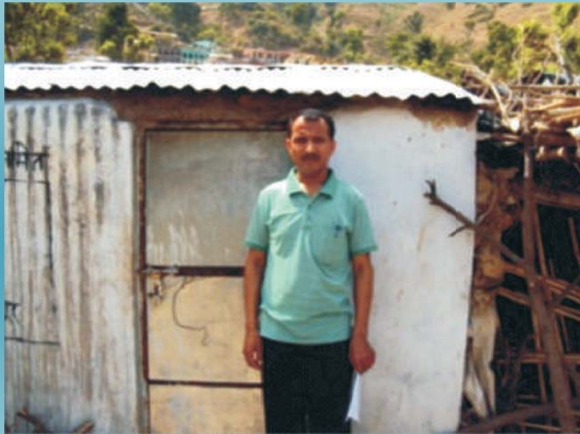
IAY house in Gaid GP, Jaunpur block of Tehri Garhwal district in Uttarakhand (Year of sanction:2011-12) (DOP 27.05.2013)
